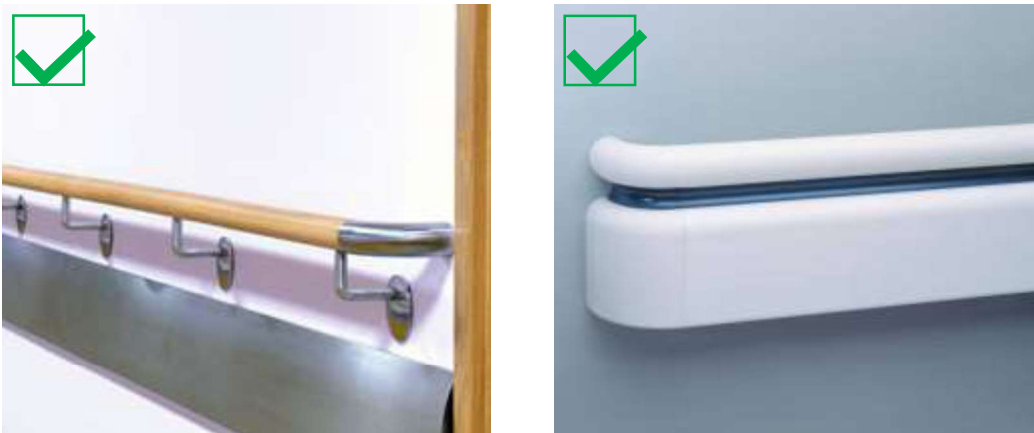
Figure 6.2: Compliant handrail examples
