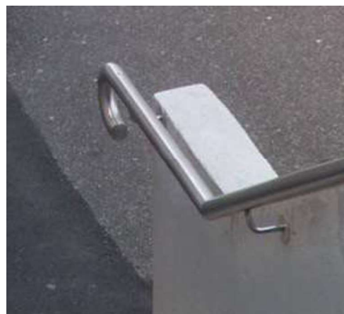
Figure 6.6: Rail extends beyond the stair.
